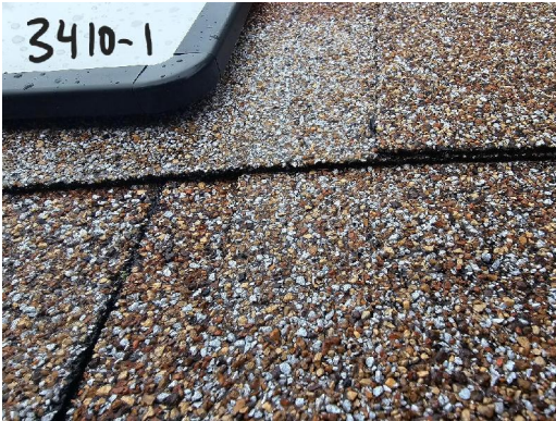
3410-1 Asphalt Shingle/Tar Typical Exterior Roof
