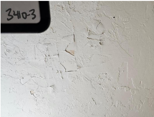
3410-3 Surfacing Texture/Tan Typical Interior Walls/Ceilings
